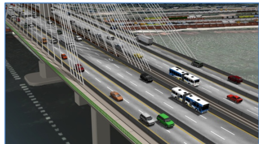
The new Port Mann Bridge will have HOV lanes in both directions for use by carpools and transit, as well as a 3metre-wide, barrier separated multi-use path
