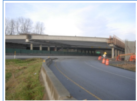
The new Kensington Avenue overpass girders being installed.
