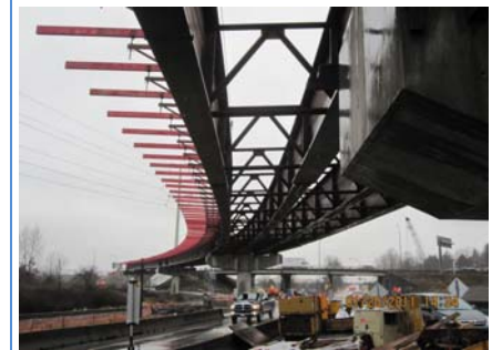
New on-ramp connecting Highway 1 to Lougheed Highway.
