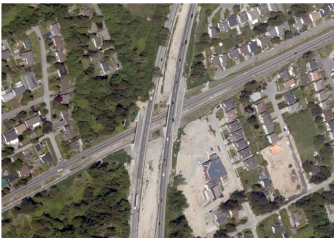
Existing 156 Street underpass at Highway 1.
