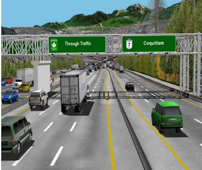
An artist's rendering of the three through-traffic lanes and two local-connection lanes approaching the new 10-lane Port Mann Bridge.
