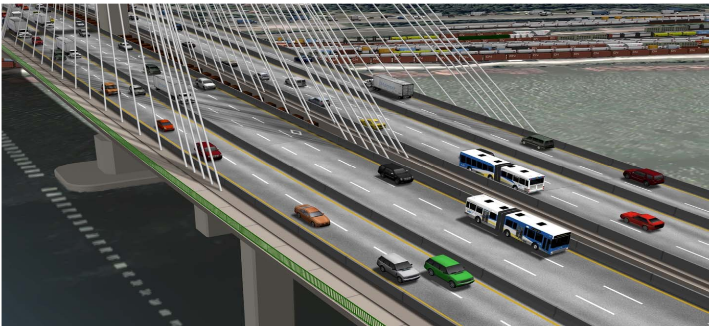
Artist's rendering of the new Port Mann Bridge with through-traffic and separated local-connection lanes as well as a cycling and pedestrian path on the east side of the bridge.
