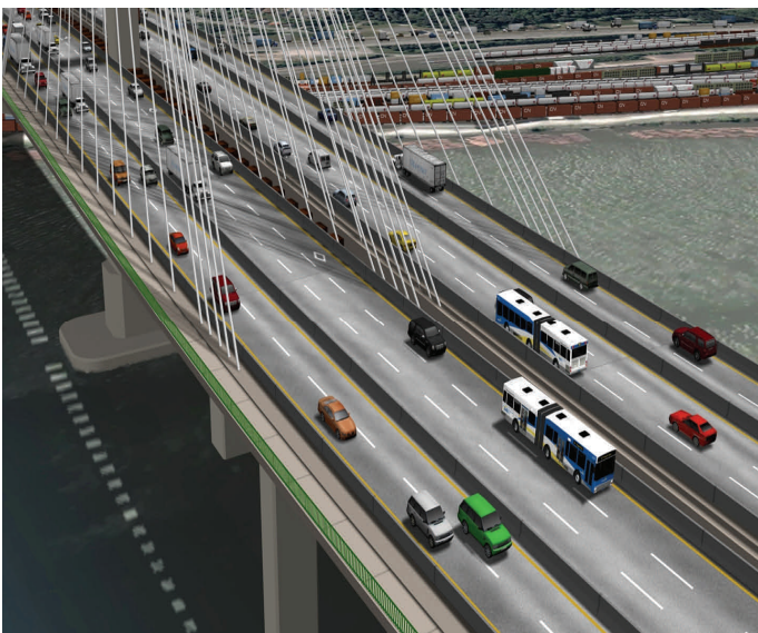
An artist's rendering of the completed Port Mann bridge, with local connection, through and HOV lanes as well as RapidBus service and a multi-use pedestrian and cycling path running across the bridge.
